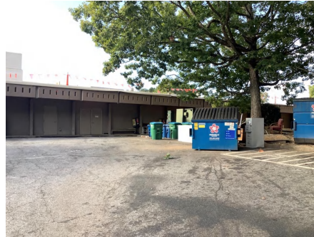
2). North Elevation - Dec 04, 2019
