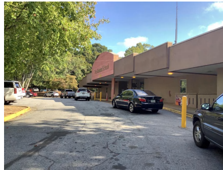
5). Southwest Elevation - Dec 04, 2019
