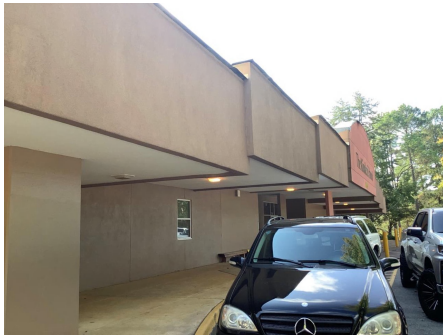
4). West Elevation - Dec 04, 2019
